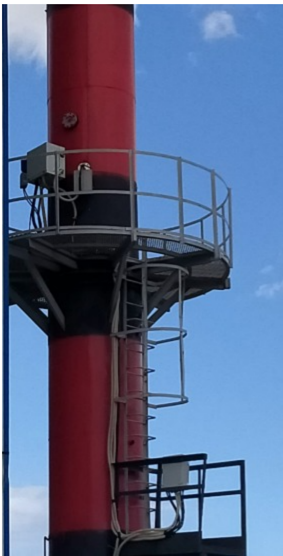
Figure 3.3 – Installation of sensors on emission tubes
